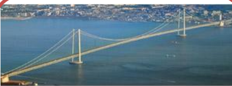
A Suspension Bridge is usually built using: steel cables and reinforced concrete
