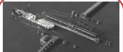
A Swing Bridge pivots on the center pillar to allow passage
